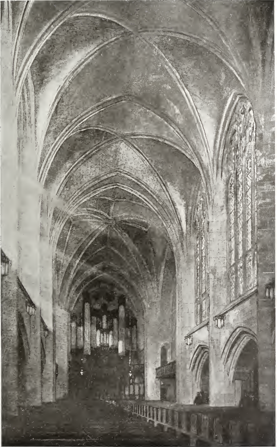
INTERIOR—FIRST BAPTIST CHURCH. Pittsburgh, Pa. New York Office, 1909.
